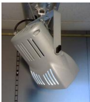
"Ioduri" reflector with 150 W discharge bulb
